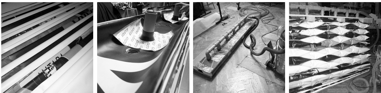
Figure 5: Process of prototyping: cutting and joining banners - connecting to inflatable device - preparation of supporting structure - inflating the prototype.
